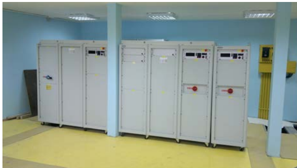
Fig. 5. Power supply system for magnets and lenses
