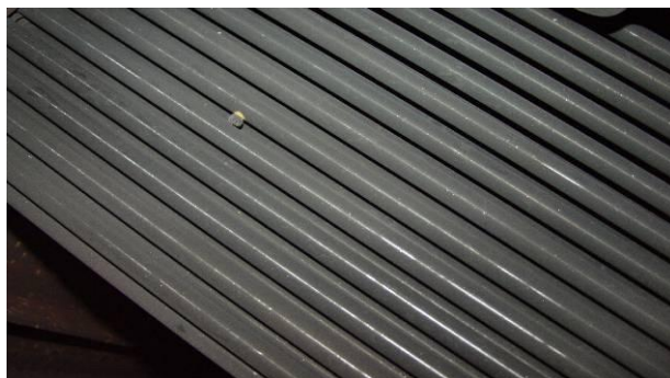
Fig. 7. HET PGV-1000M power unit No 3 Rivno NNP (start-up 1986), Chemical cleaning SG was provided periodically from 1998 to 2007
