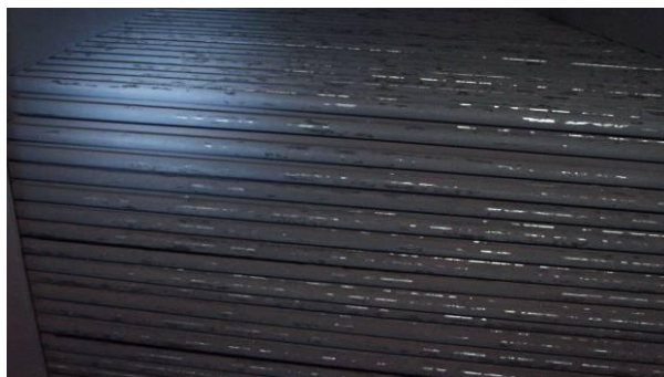
Fig. 6. HET PGV-213 power unit No 1 Rivno NNP (start-up 1981), Chemical cleaning SG not provided
