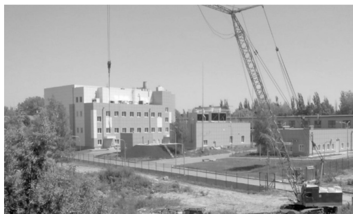
Fig. 7. The building of the Neutron Source Facility under construction in Kharkiv (© SSTC)
