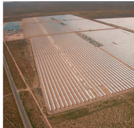
Figure 6. Aerial view showing portions of Solar Energy Generating Systems (SEGS) (California, USA).
