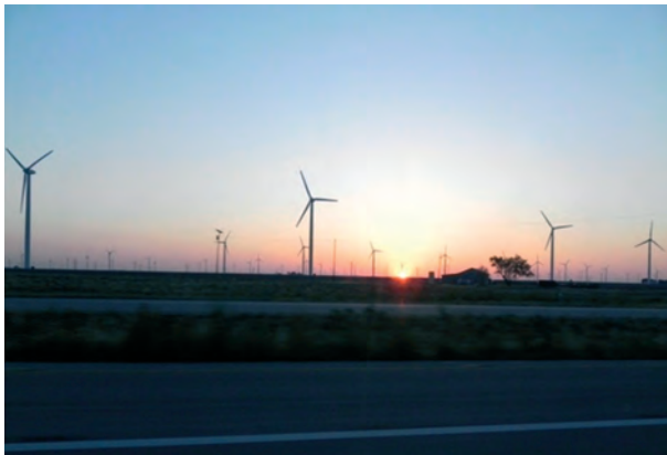
Figure 5. Second largest in the world 781-MW el onshore Roscoe wind-turbine power plant (Texas, USA).
