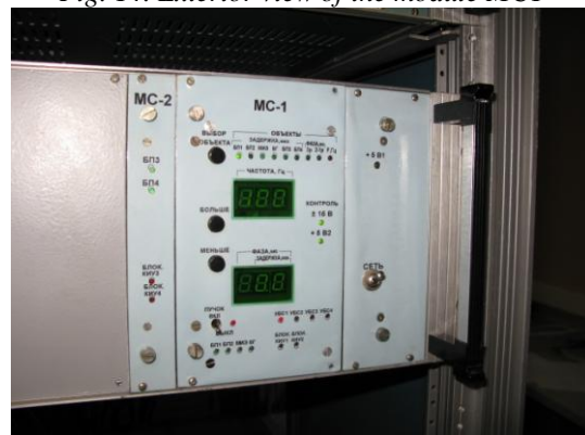
Fig. 15. Exterior view of the synchronizer accelerator LU-60M
