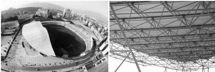
Fig. 2. The membrane roof of one stadium
