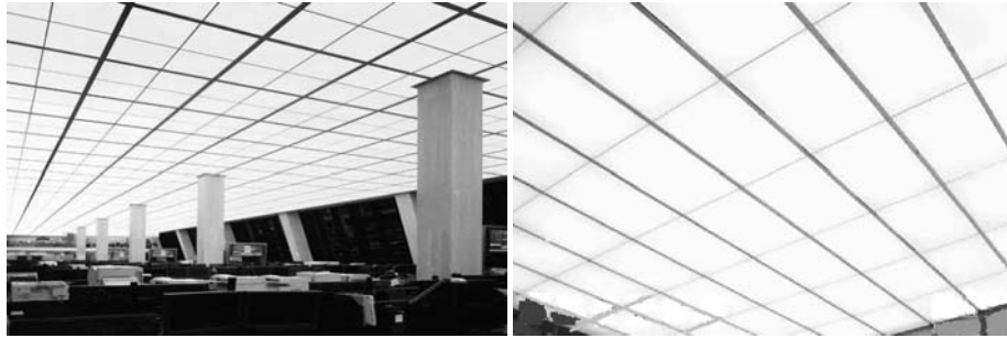
Fig. 1. The membrane roof of one office building
