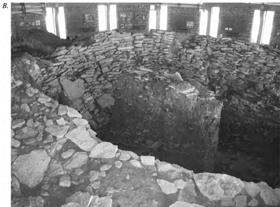
Fig. 12. The stone construction from Cucuteni–Gosan, Tumulus 3. A. Drawing after Dinu, 1995: 121, fig. 2. B. Photograph of the actual state of preservation of the tomb, inside a museum.
