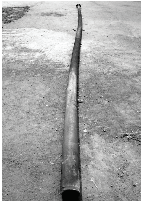
Fig. 1. Photography of the failed tube.
