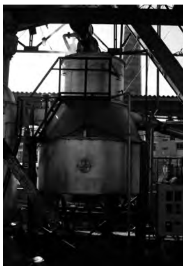
Fig.3. 3 MW generator at Malin paper factory.
