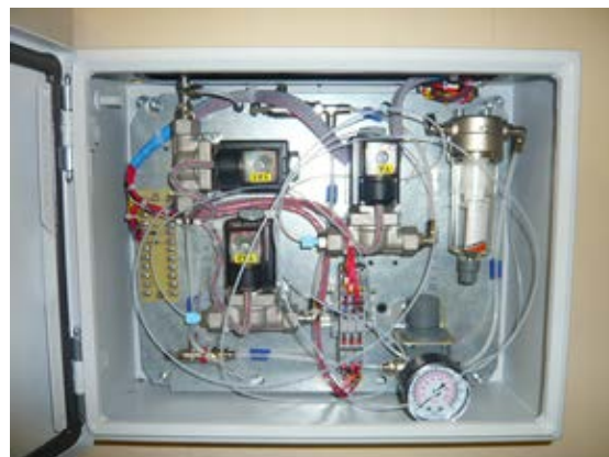
Fig. 9. The unit for filling the target with nitrogen for ^{11}\text{C} production
